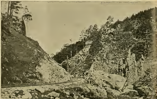
NATIONAL RAILWAY ENTRANCE TO THE BARANAS OF THE PINO (THREE PINO).
